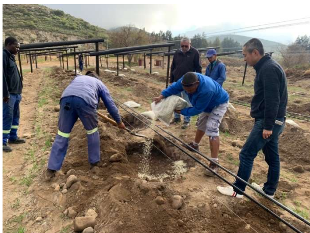
Application of Porous Alpha at a farm in South Africa
